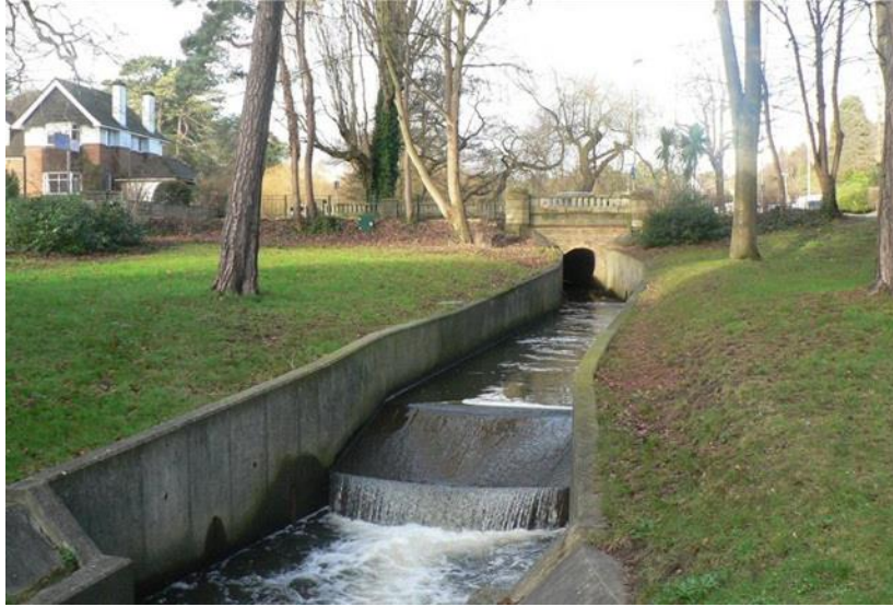
Chris Downer / Bournemouth Gardens: concrete channel
